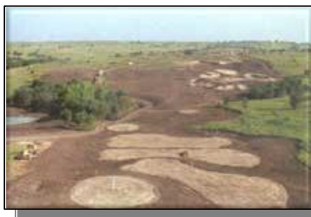
The construction of Colbert Hills Golf Course near Manhattan, Kansas.
