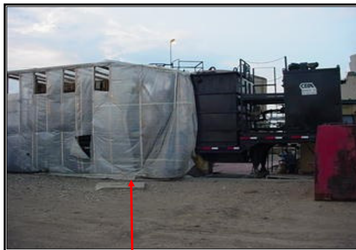
Preparation/loadout of Clarified Slurry Oil (CSO) hazardous waste for shipment to DGC plant
