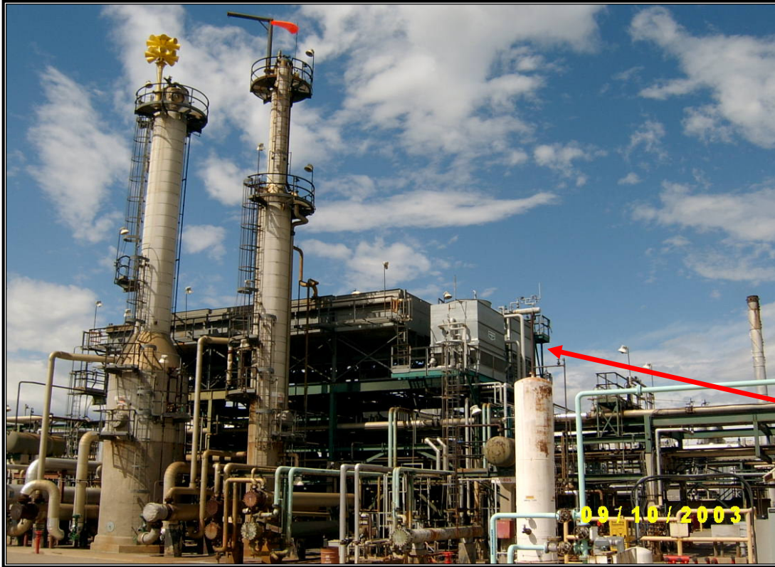
Ammonia adsorption refrigeration unit
