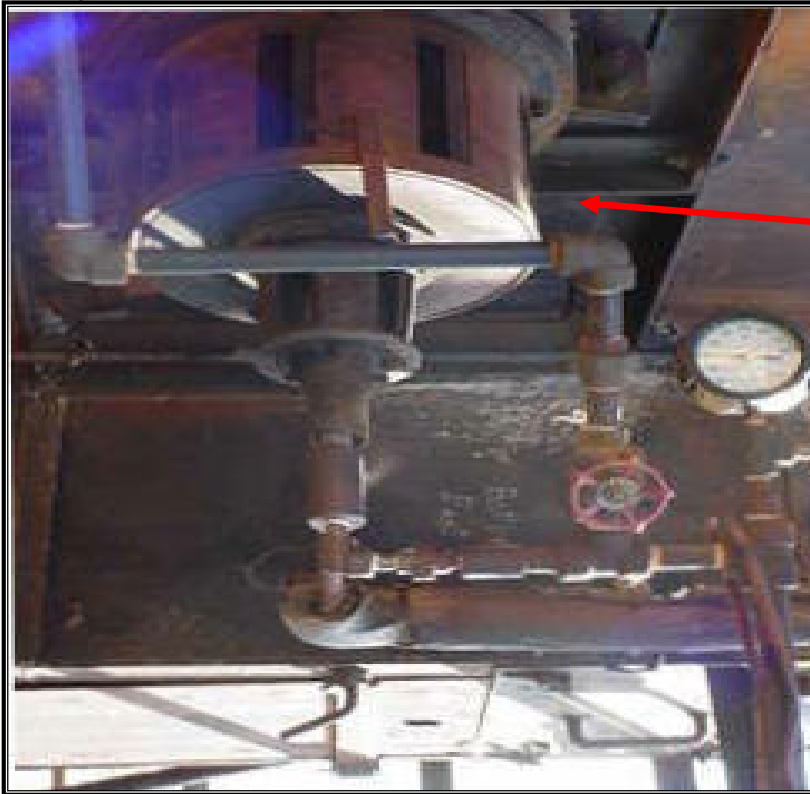
Heater burner/inlet assembly modified for Acid Soluble Oil (ASO) combustion. ASO is a unique and complex mixture of waste oils generated during the alkylation process. ASO has significant Btu
