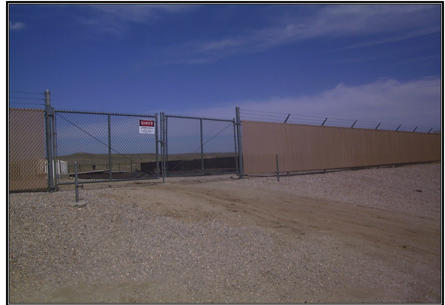
Wastewater management areas designed to minimize storm silt inflow. Slats in fence can reduce added waste volumes by a surprising 20 - 30 % in areas such as Wyoming.
