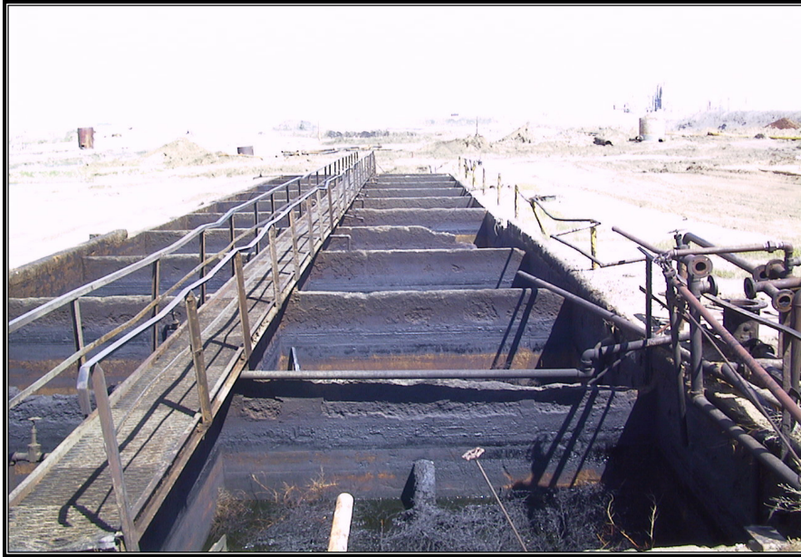
Wastewater management areas open to windblown particulate, storm silt, etc. can surprisingly add to oily waste generation with accumulation of these solids in units.
